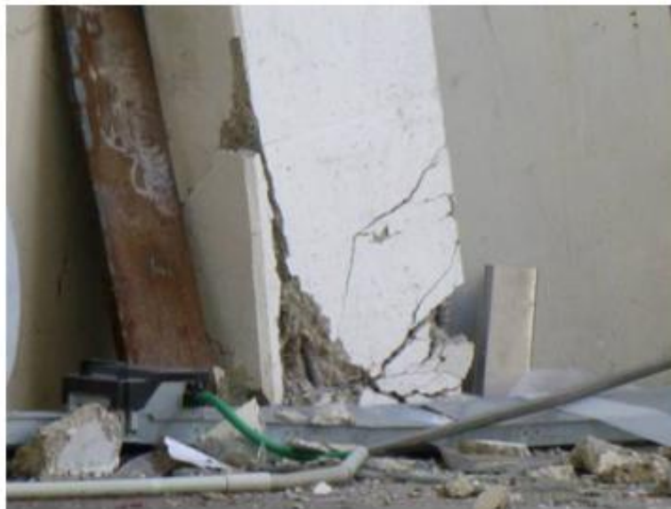
Figure 1 Formation of a plastic hinge at the base of a column (Figure adapted from [10])
