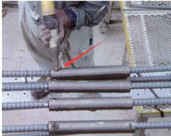
Figure 21 Sleeve grouting connection (Figure from [21])
