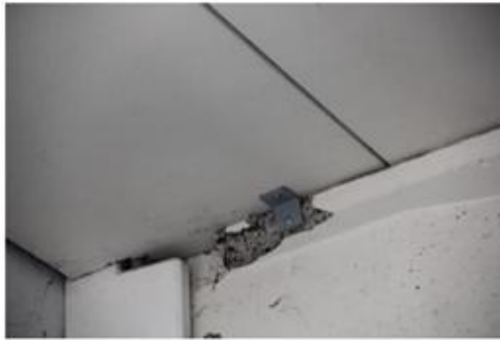
Figure 6 Inappropriate beam-to-roof connection (Figure adapted from [9])
