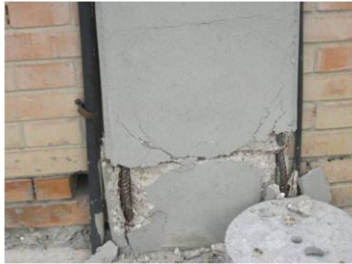
Figure 2 Buckling of longitudinal rebars at the base of the column (Figure adapted from [10])
