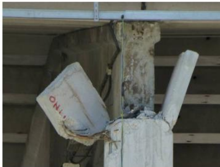
Figure 4 Failure of lateral restraints of the pocket support. (Figure adapted from [10])
