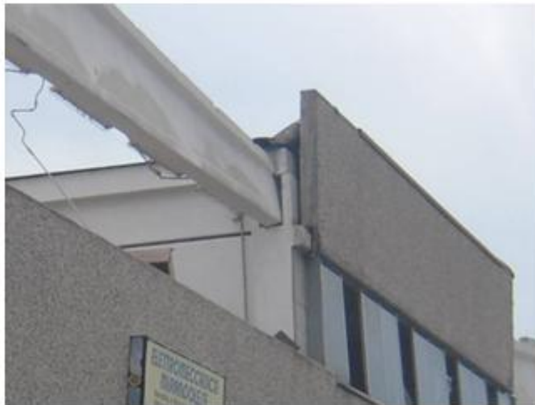
Figure 5 Out-of-plane counterclockwise rotation of the shed beam, and clockwise rotation of the cladding panel (Figure adapted from [10])
