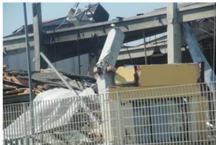
Figure 3 Short column effect derived from presence of the masonry infill walls (Figure adapted from [9])
